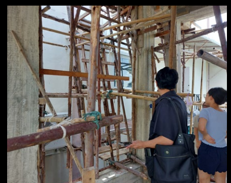
BAMBOO USED AS IMPROVISED SCAFFOLDING, PROPS AND LADDERS.
