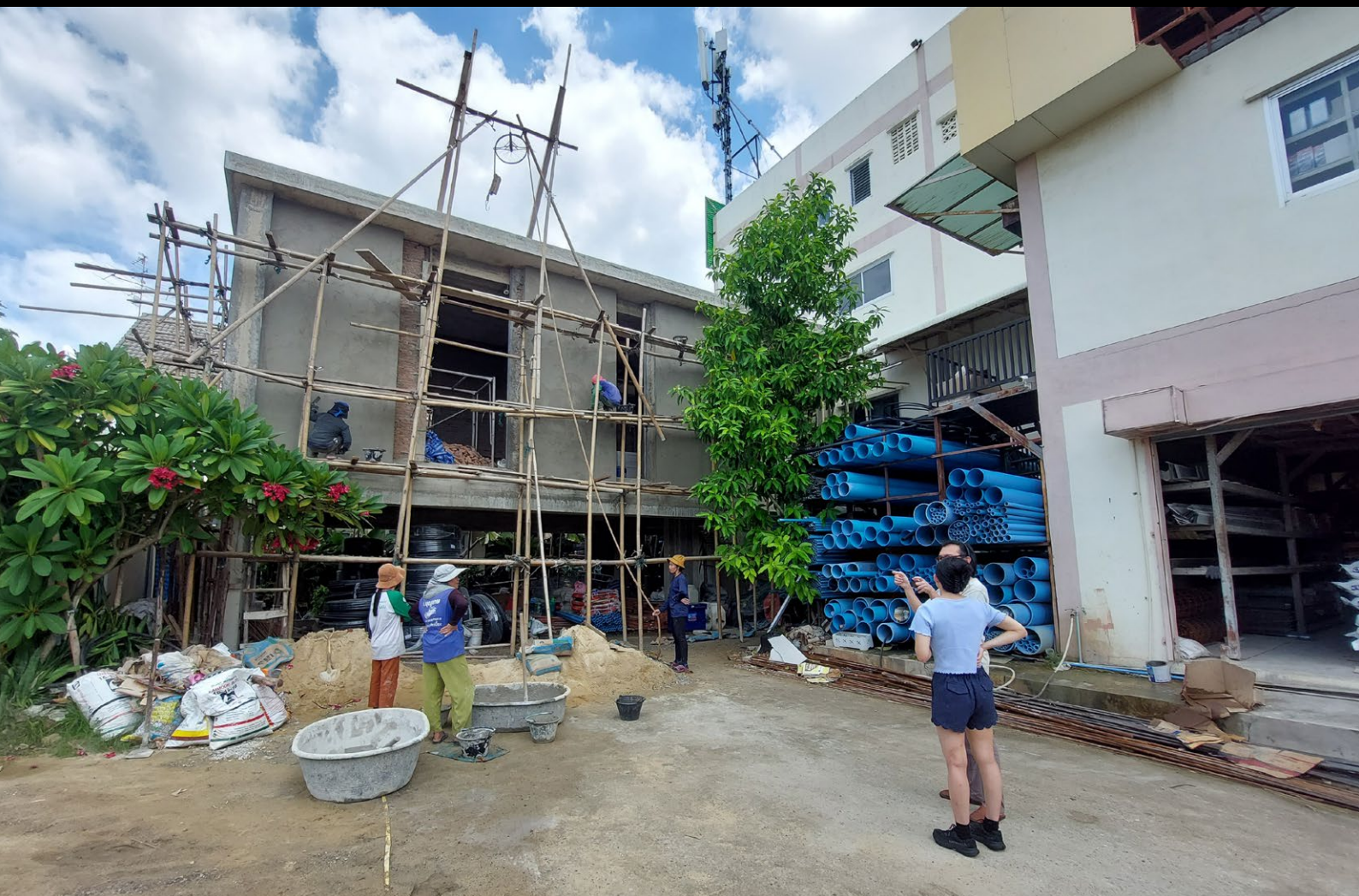
LAM AT THE GAI KAI RECORDING STUDIO A CONSTRUCTION SITE.
