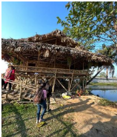
Figure 2: Front view of the structure
