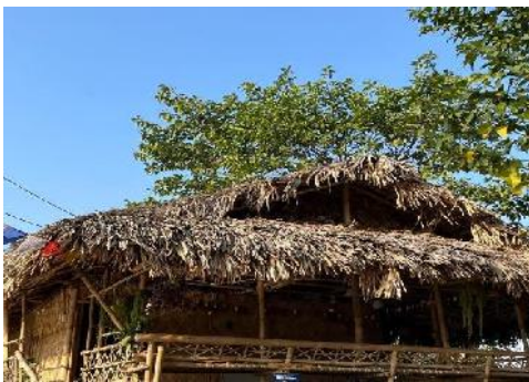
Figure 6: Roofing of Bamboo House
