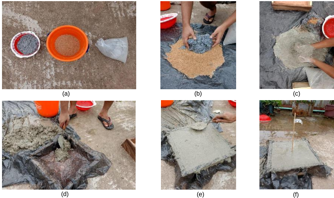
Figure 6: (a)Arranging materials–paper,sand,cement, (b-c)Mixing, (d)Filling up the mould, (e) Seamless papercrete filling, (f) Adding Label
