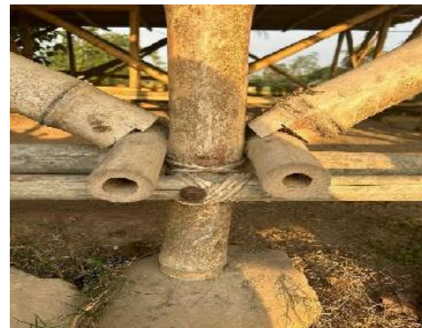
Figure 9: Nut and Bolt Joint
