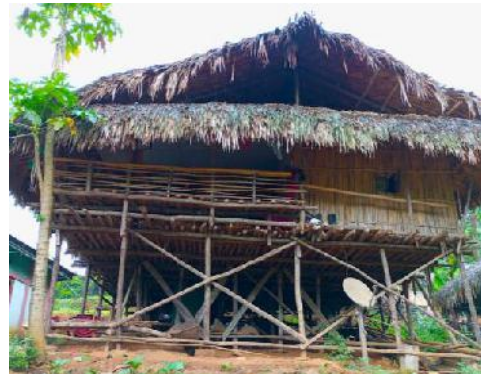
Figure 1: A Bamboo house in Arunachal Pradesh
