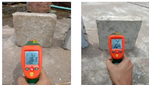
1 2 Time:12.30 P.M (1.Outer facade 2.Shaded facade)
