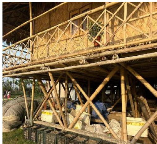
Figure 3: Side view of the structure
