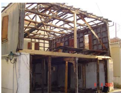
FIGURE 19: Timber Frame independent from the masonry infill (Karababa & Guthrie 2007)
