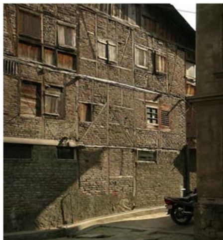
FIGURE 11: Dhajji-Dewari System (Hicyilmaz et al. 2011)
