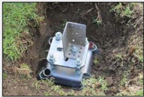
Figure 4.8 (a): Footing plate with 4 guide tubes on the corners of the plate at angles away from the centre (SF150)
