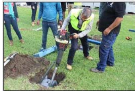
Figure 4.8 (b): "SureFoot" footing installation during the study project at Burnley Campus of the University of Melbourne
