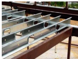
Figure 4.10 (a): Galvanised cold-formed metal decking system for durability
