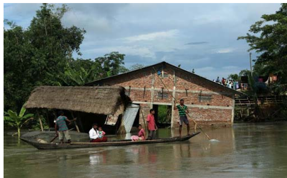
Fig. 2.1 (b): Flood inundation and damage to houses in rural Assam ( source: Flood Report Assam)
