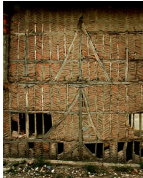
FIGURE 7: Himis type of construction (Gulkan 2004)
