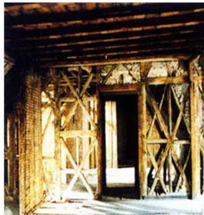
FIGURE 18: Gaiola timber frame (Cardoso et al. 2004a)
