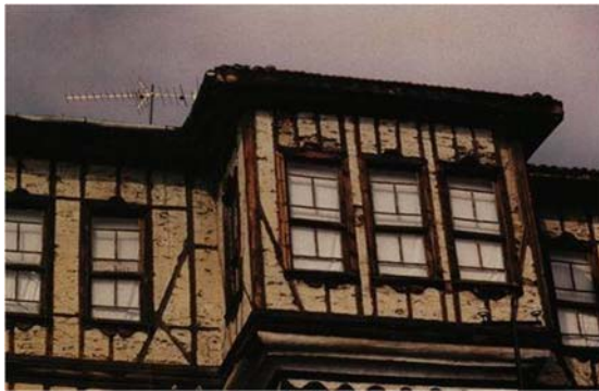
FIGURE 12: Bagdadi construction in Turkey structure (Ozturk & Chantimur 2011)
