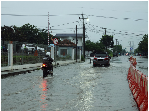
Figure 2. Water ponding on several roads in Gedebage after heavy rain. Image by Asep Darmana.
