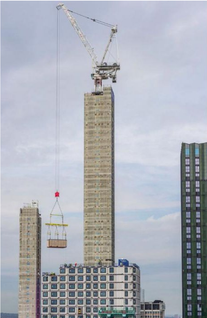
Image 21: College Road module lift
