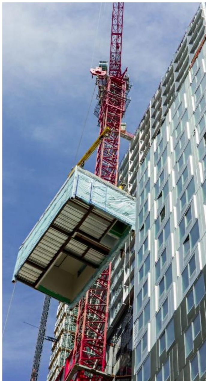
Image 20: 461 Dean Street module lift
