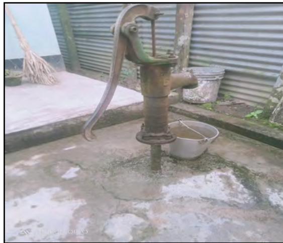
Figure 9: A tube well, another major source of water
