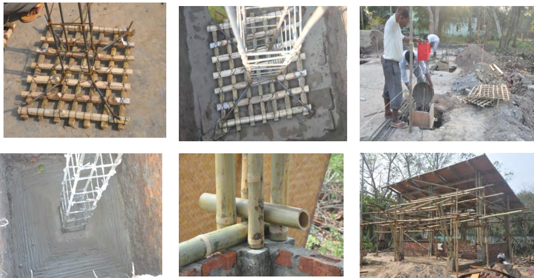
Figure 15: Bamboo reinforcing mat in RFRI, Jorhat (Courtesy: R.Kalita)
