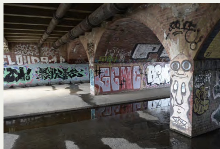
The bridge under a bridge. An open air gallery.
