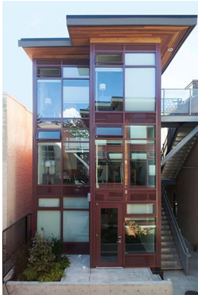
Figure 2: Social housing built from converted shipping containers in Vancouver (Photo source: Atira Women's Resource Society )
