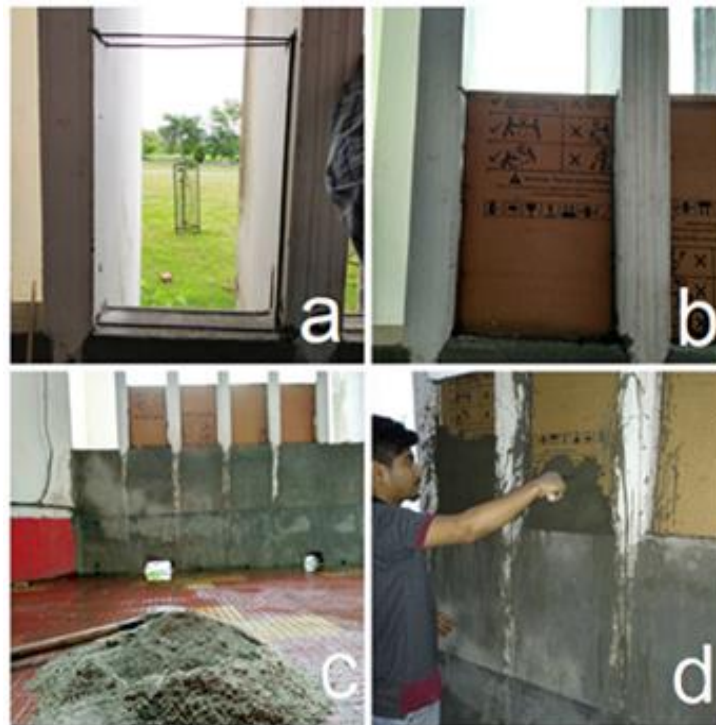
Figure 3: Construction of cast-in-situ wall panels using a. scrap rebars for making frame, b. Cardboard back-support behind wire-mesh, c. Mortar for base-course, and d. Placing of mortar on wire-mesh against back support.
