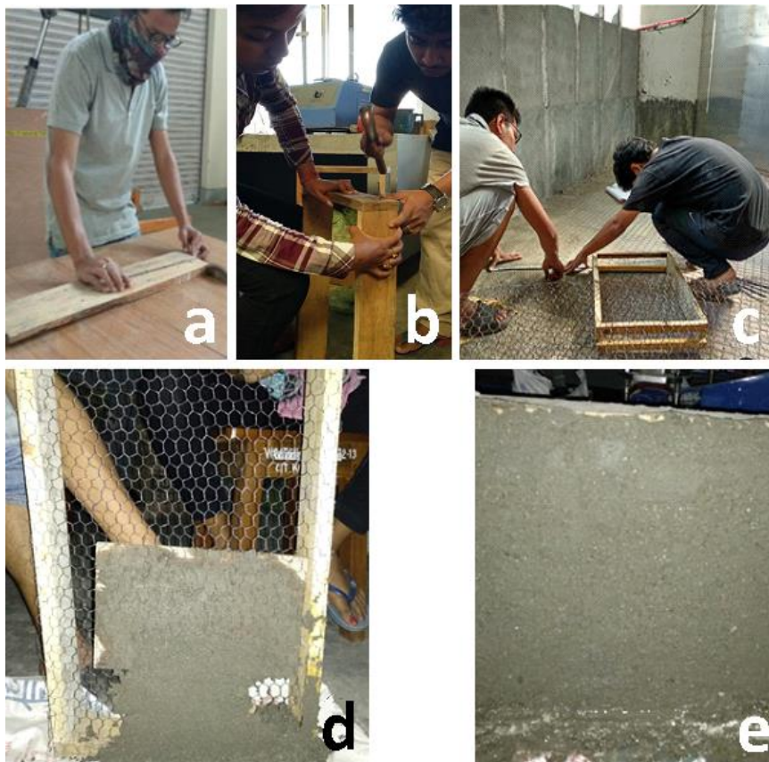
Figure 2: Materials for construction: a. preparation of timber pieces for making frame, b. making frame, c. fixing wire-mesh on the frame, d. applying mortar on wire-mesh for the base-course, e. competed base-course of the panel.
