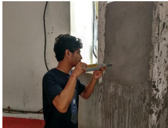
Figure 5: Rebound hammer test on ferrocement panels of cavity wall
