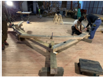
Carpenters and apprentices setting out timber frame, Nivillac, France. Source: Author, 2022.
