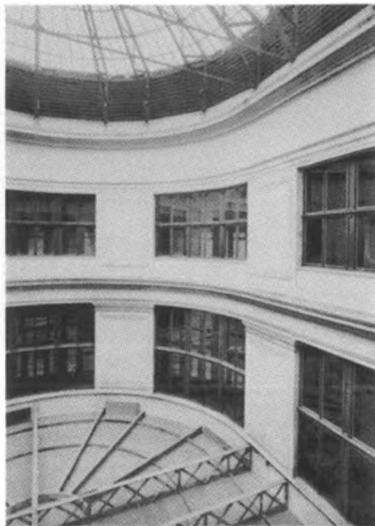
O Wagner: Länderbank, view of light well above the banking hall, Vienna 1884, phot: J Dapra
