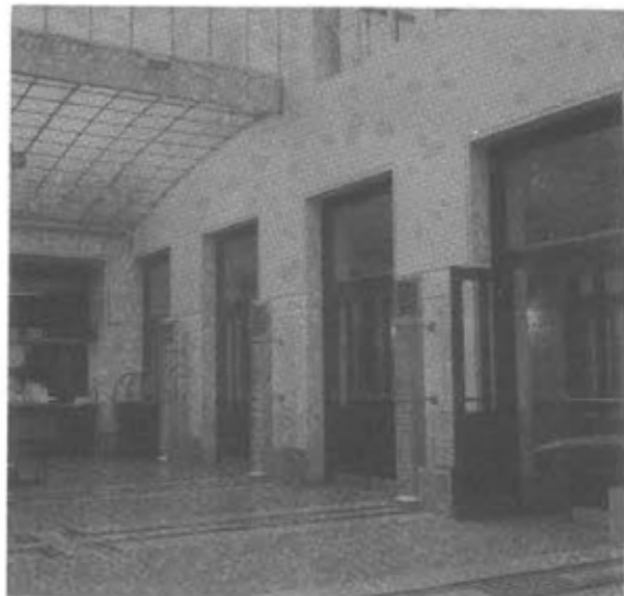
O Wagner: POSB, contemporary view of entrance to banking hall, phot: R Wolff
